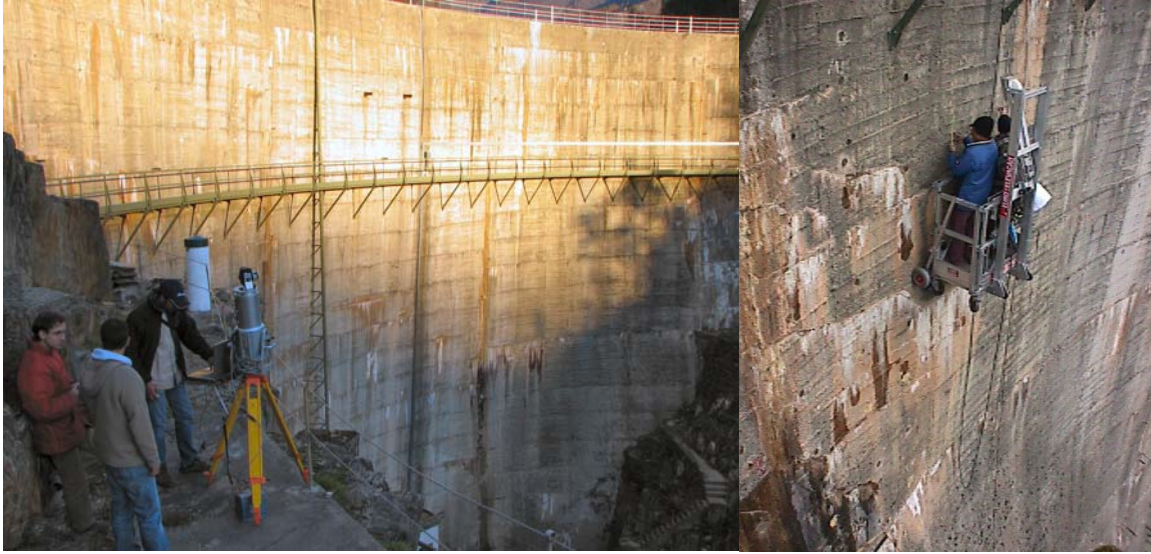
Fig. 1. Downstream face of Alto Ceira dam and laser scanning inspection.
