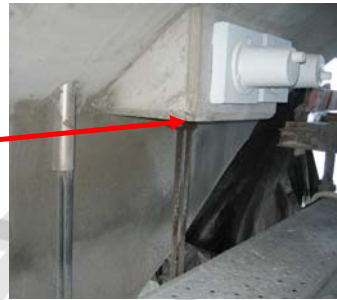
Piers P7 and P10 - Anchorage of the deck to the piers
