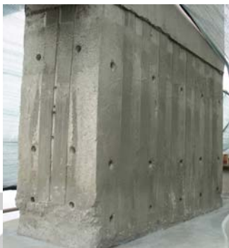
Pier strengthening - Fiber anchorage zones
