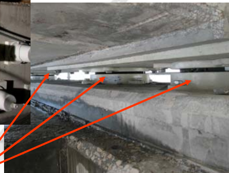
Substitution of bearings
