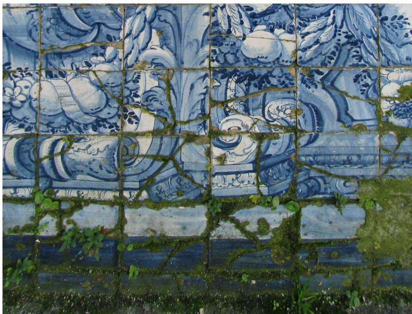
Figure 1- Decaying panel in a now exposed area (Oporto Cathedral, upper cloister gallery)
