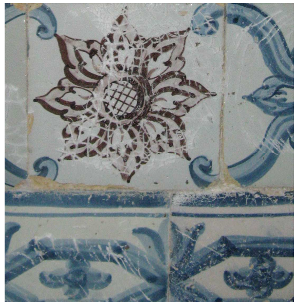
Figure 3b- Efflorescence at the same panel
