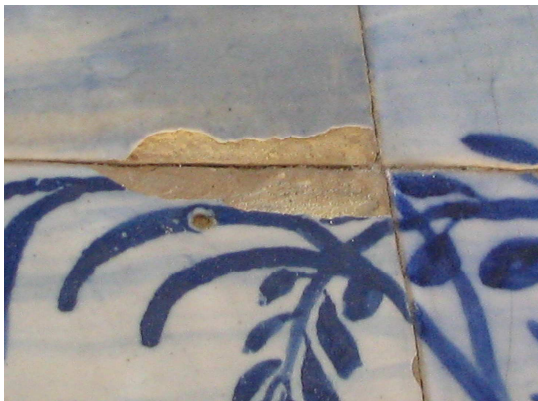
Figure 5- Decay progressing from edges
