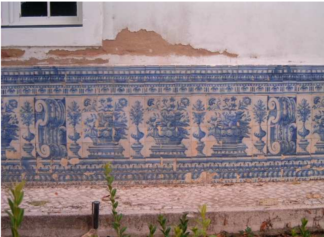
Figure 2- Salt crystallization above a street azulejo panel at Casa dos Patudos (photo by Manuel Anastácio, Wikimedia)
