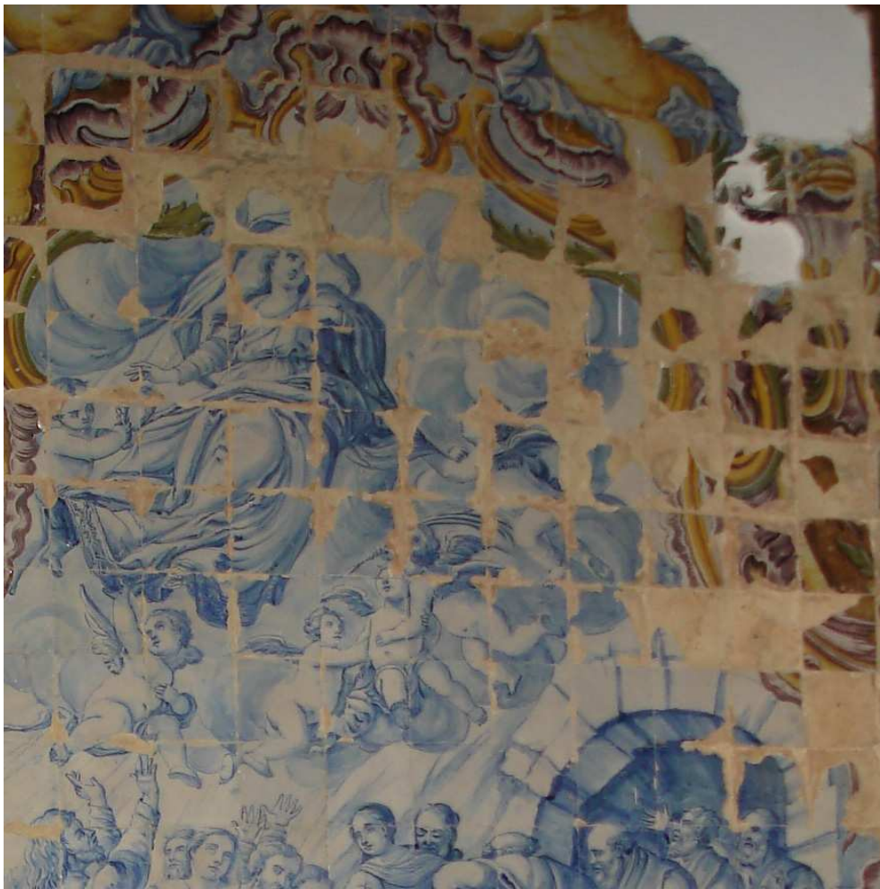
Figure 4- Generalized decay at the wet zone of an interior panel (Church of Jesus, Setubal)
