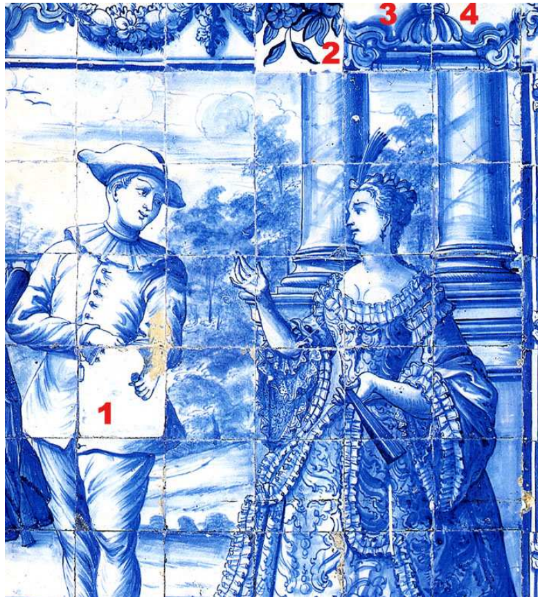
Figure 6- Panel with four missing azulejos reintegrated with replacements at an undetermined date [4]
