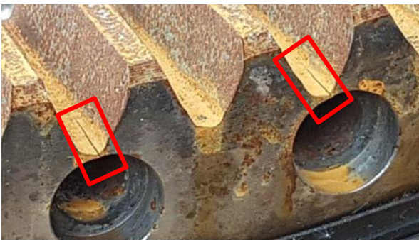
Fig. 11 | Detail of the rack where two fractures are identified.
