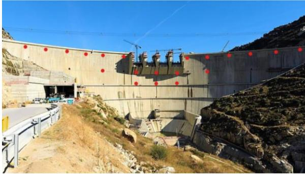
**Fig 6** - Accelerometers position on the vibration-based monitoring system (marked with red dots)
