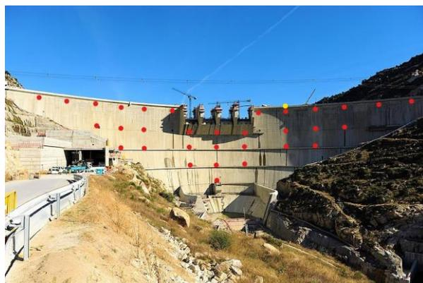
**Fig 4** - Vibrator and accelerometers position during forced vibration tests
