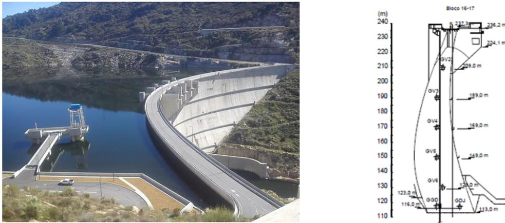
Fig 2 - Baixo Sabor arch dam with full reservoir [5] and cross-section through the central cantilever
