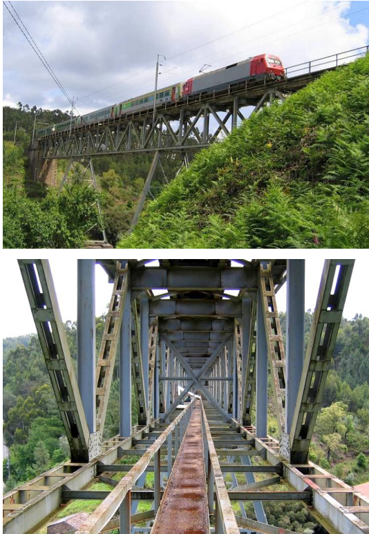
Fig. 3 - Trezói bridge: (top) lateral view; (bottom) view inside the deck.
