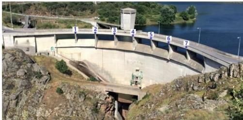
Fig 9 - Caldeirão dam: test layout
