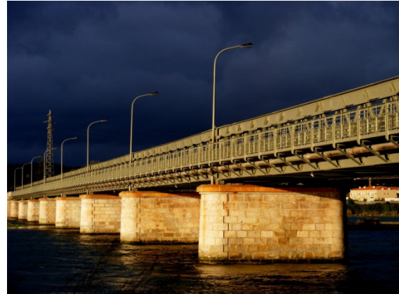
Fig. 1 – Global overview of the Fão Bridge.
