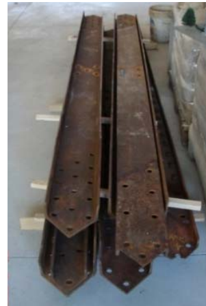
Fig. 2 – Diagonals removed from the Fão Bridge.
