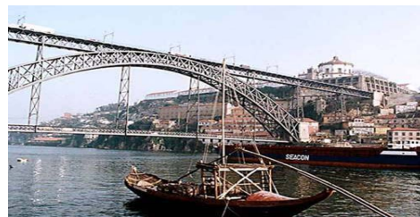
Fig 1a - Highway Luiz I bridge.
