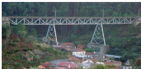
Fig 1d - Railway Trezói bridge.
