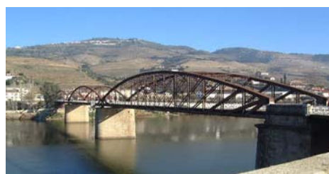
Fig 1b - Highway Pinhão bridge.
